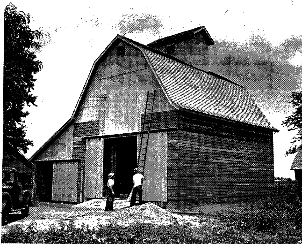
Figure 33. Farm families built many new corn cribs in the 1940s and 1950s to deal with increased yields due to hybrid seed, fertilizer, and pesticides. Cribs like this one in Washington County were built to hold ear corn harvested by mechanical pickers. Changes in harvesting soon made these cribs obsolete. Wallaces' Farmer and Iowa Homestead , 6 August 1955.
