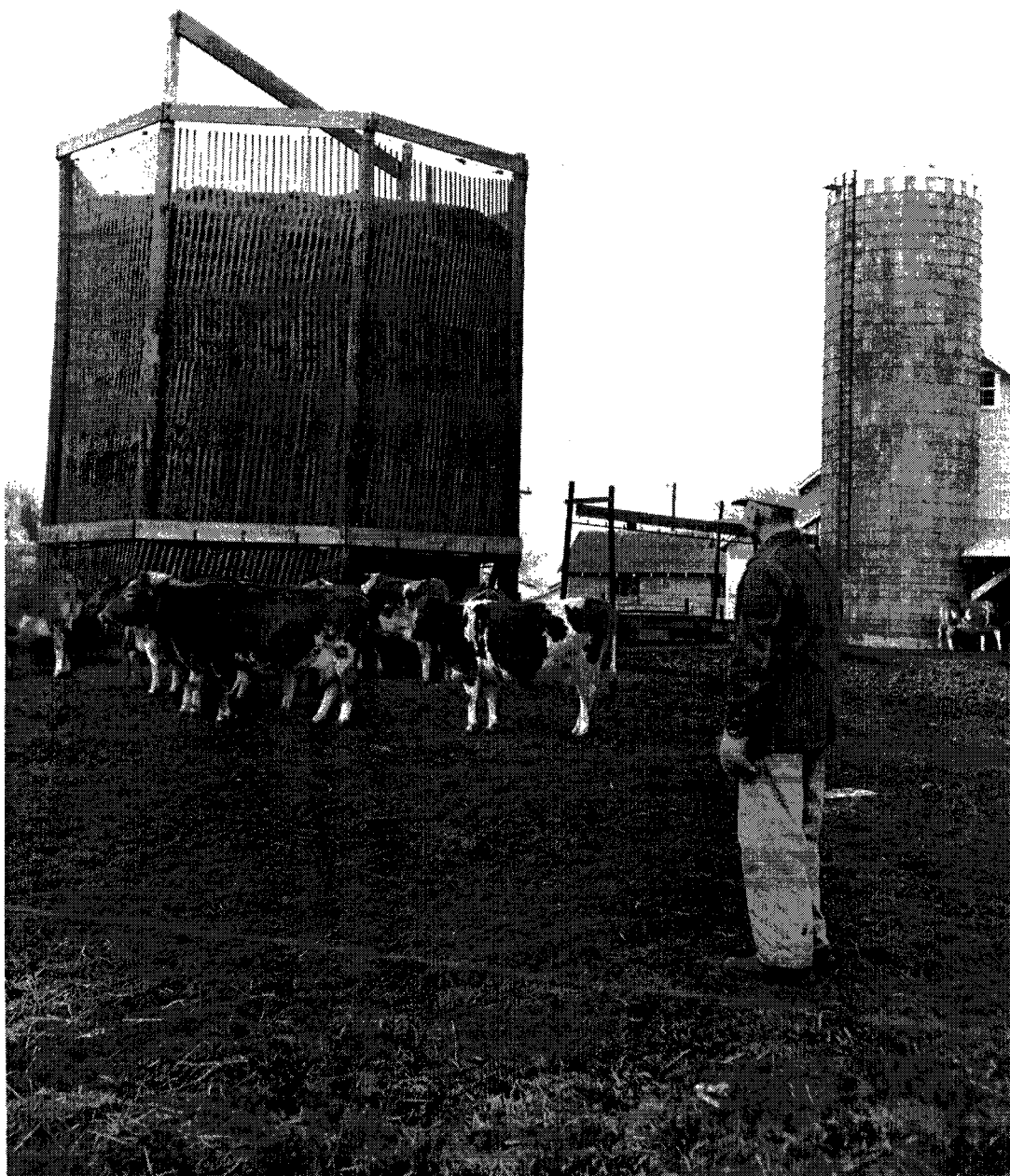
Figure 28. Self-feeding haykeepers, designed at Iowa State College, permitted farmers to cut labor costs by reducing the amount of feed they handled for beef and dairy herds. This 1956 photograph of a dairy farmer, cows, and haykeeper is from Carroll County. Wallaces Farmer .
